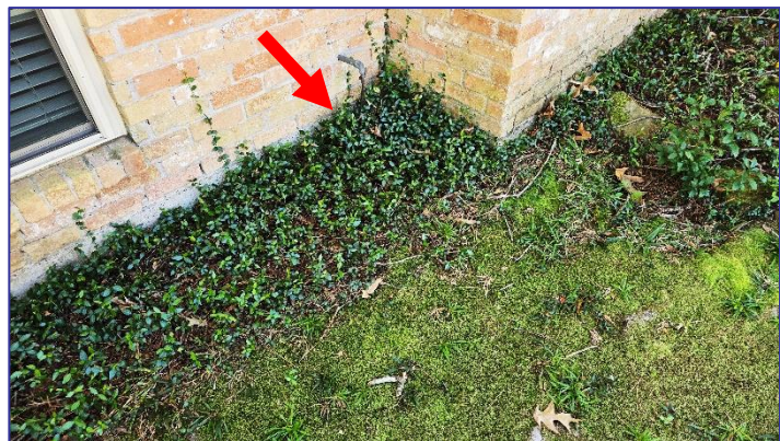
SOIL AND GROUND COVER COVERING 1 ST ROW OF BRICKS
