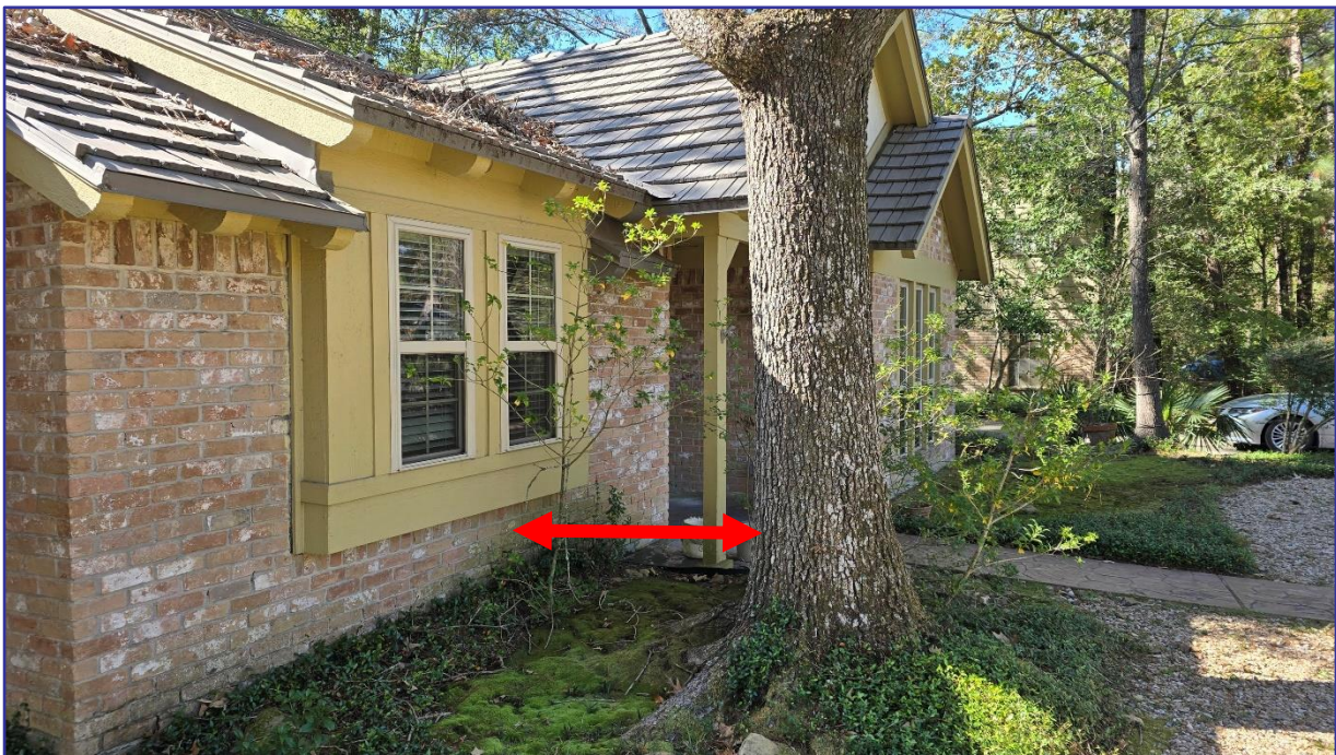
TREE CLOSE TO FRONT OF HOUSE
