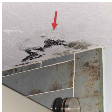
Primary Bathroom - possible microbial growth
