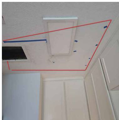
Kitchen - most affected area
